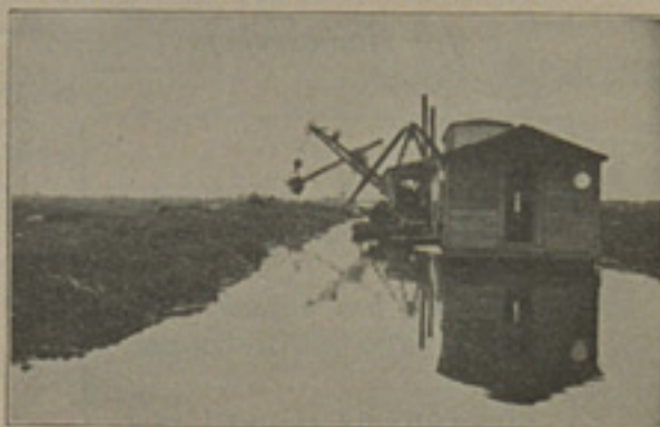
One of our dredges cutting Royal Glade Canal
