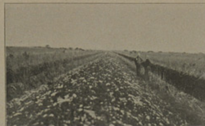
Partially completed dike along west side of Davie Farm. Since this picture was taken, the dike has been reinforced by material from a third dike.
