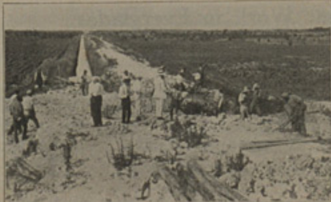
Washington Avenue, north side of Davie Farm in the Everglades. Preparations being made for the collection canal which will conduct drainage water to the pumping plants soon to be installed.
