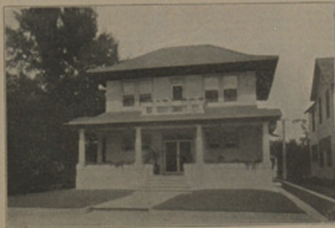
Residence of Theodore Hoffmeyer, Miami. This is typical of the fine class of homes that have been built in and around the "Magic City."
