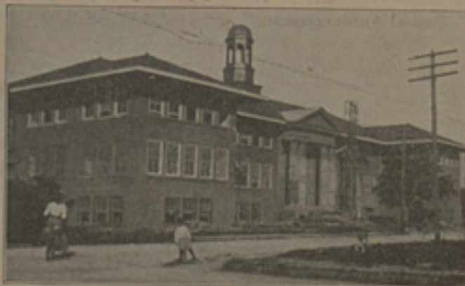
New $75,000 High School Building, Miami, Nearing Completion.
