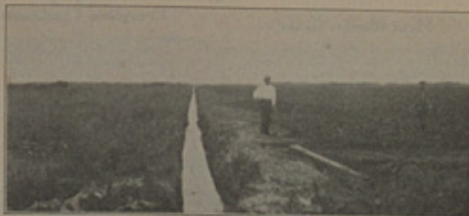
Mortenson and Wall Preparing Tract 33, Section 27, Davis Experimental Farm, for Winter Cropping. In the Foreground is One of the Many Lateral Ditchers Installed by the Everglades Land Sales Company.
