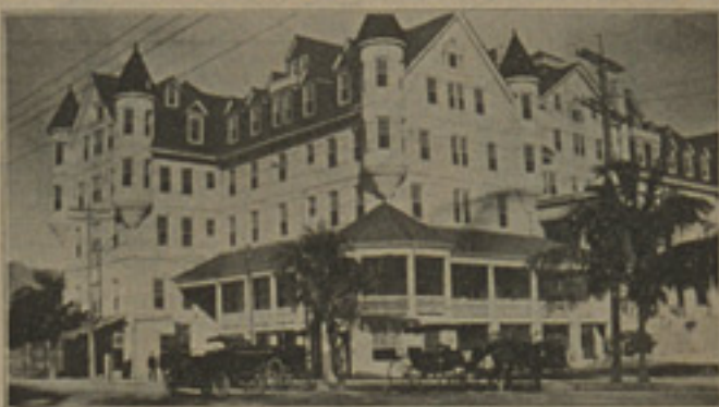
Halcyon Hall—One of Miami's Many Hostelries. This Building was Constructed from Miami Rock. Note the Beautiful Snow-white Appearance.
