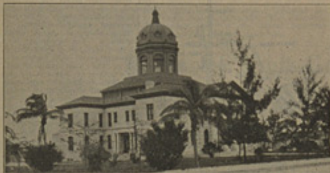
Dade County Court House, Miami. Built of Miami Rock—the Same Material from Which the Famous Dade County Roads Are Also Constructed.
