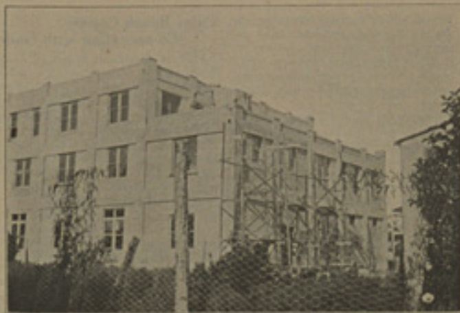
Masonic Temple (Concrete Building) Being Constructed at Ft. Lauderdale.
