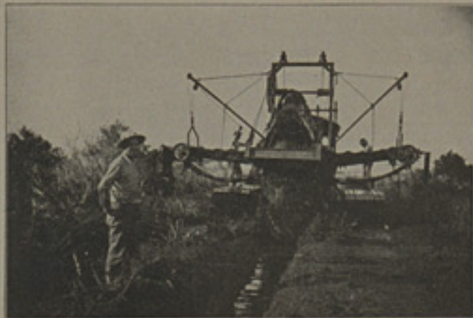
Buckeye Ditcher Cutting Ditches in the Everglades.
