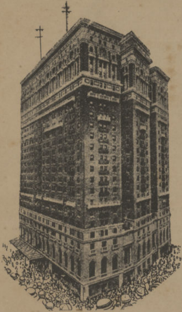
"WMCA Radio Broadcasting Station"
