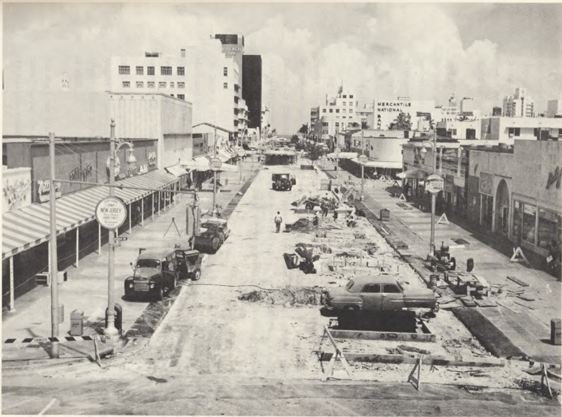
LINCOLN ROAD MALL UNDER CONSTRUCTION 1960
