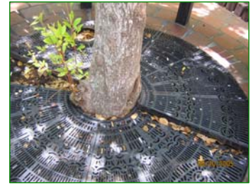
Bad Practice: Tree Grate Girdling Tree
